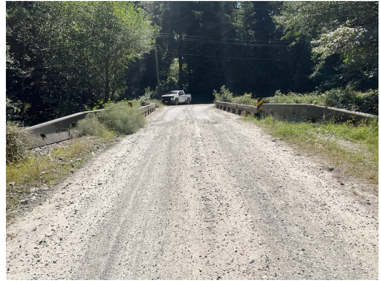
Approach from Right Bank when facing downstream
