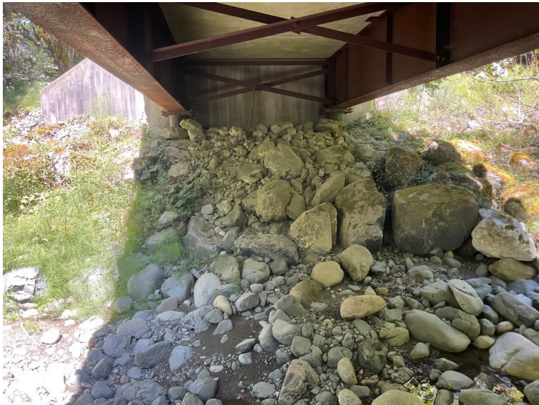
Right Bank Abutment when facing downstream
