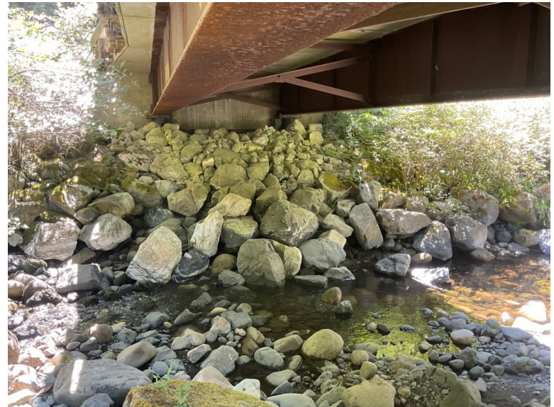
Left Bank Abutment when facing downstream
